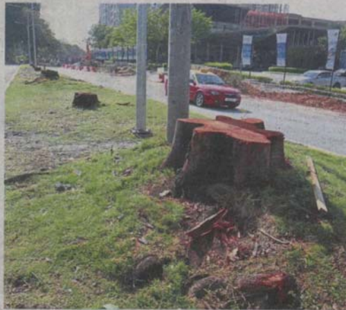
A total of 26 large trees along Jalan Universiti have been cut down to make way for road widening works.
